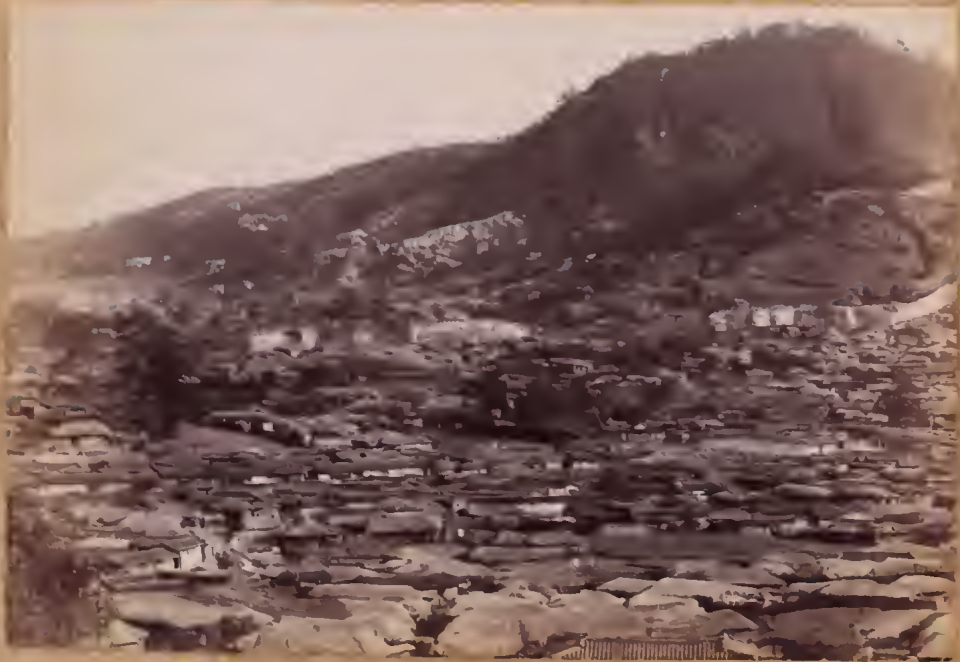
Nam Sien - the South Mt. - Inside City Hall.
